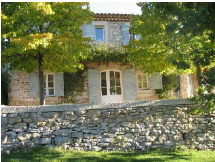
Our villa in Buoux (Provence)
